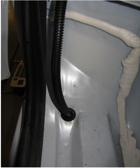
Figure 71. Wiring harness routed into cab.
