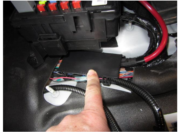
Figure 72. Wiring access under driver seat.
