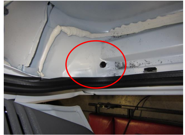
Figure 69. Access hole drilled into driver side foot well.
